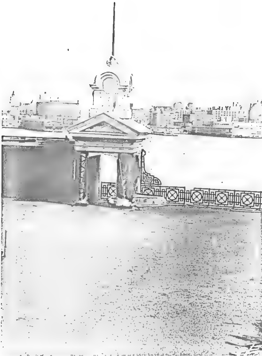
View of the southernmost belvedere at parapet of facade over ferry slips. Decorative iron railing is seen to the right.
